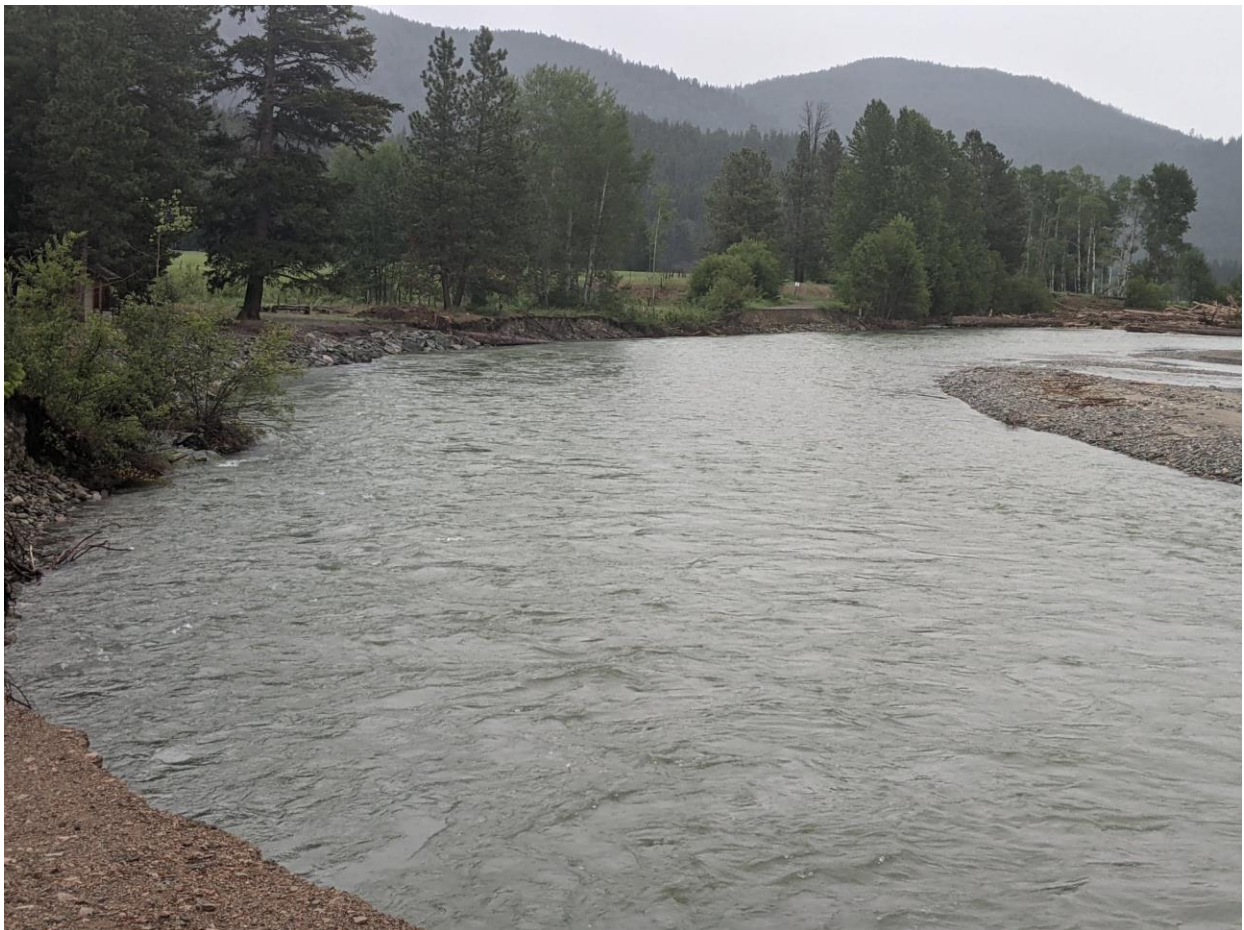
Collins Gulch Road KVR Washout
